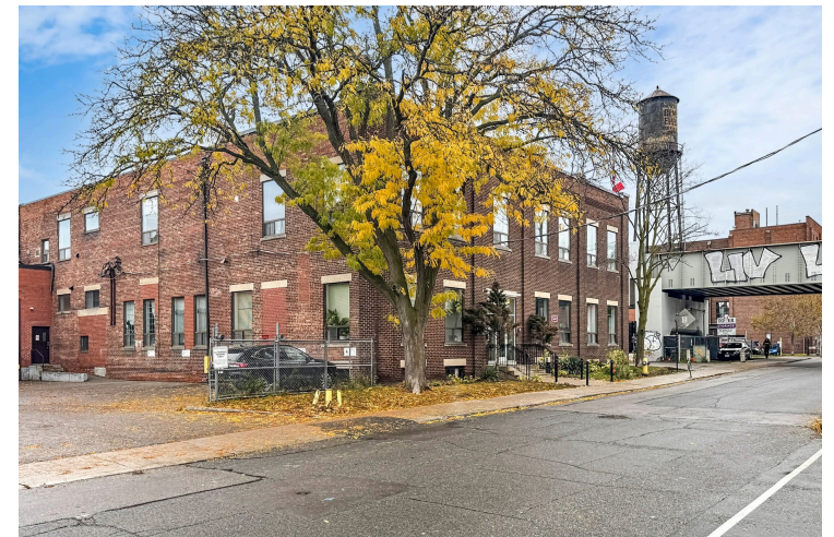
The loading dock on Wallace; the Wallace and Sarnia corner.
