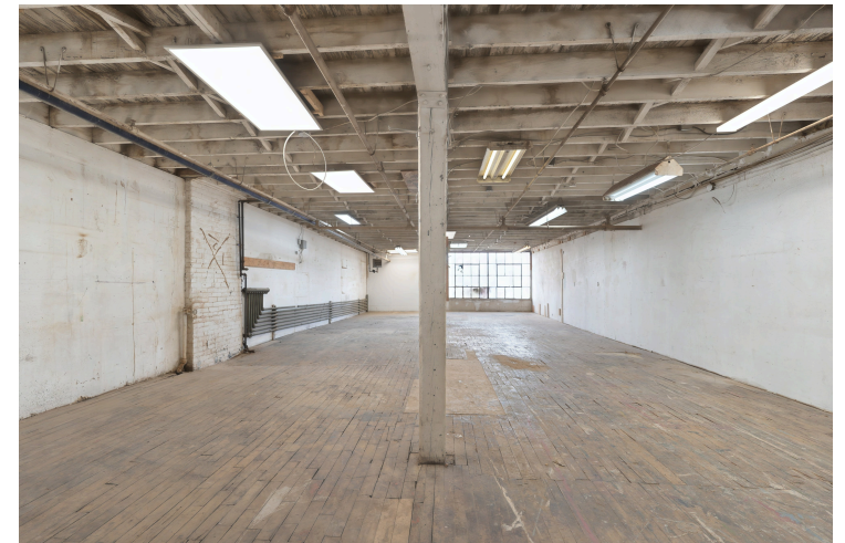
Two more views of the open floor.
